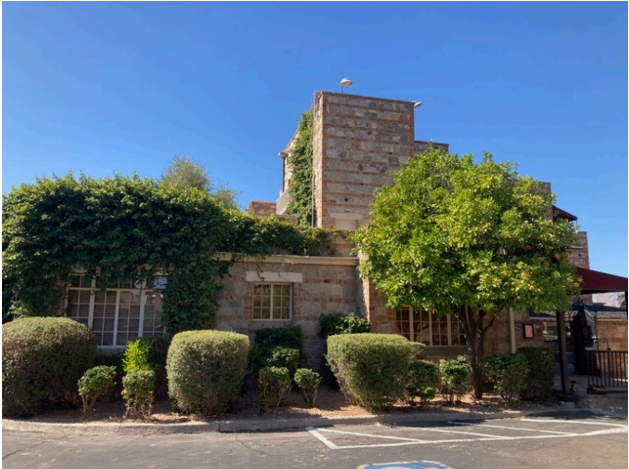
7 of 17 . AZ_PimaCounty_ElDoradoLodge_0007 South façade of the Mountain Oyster Club from parking lot. Facing North
