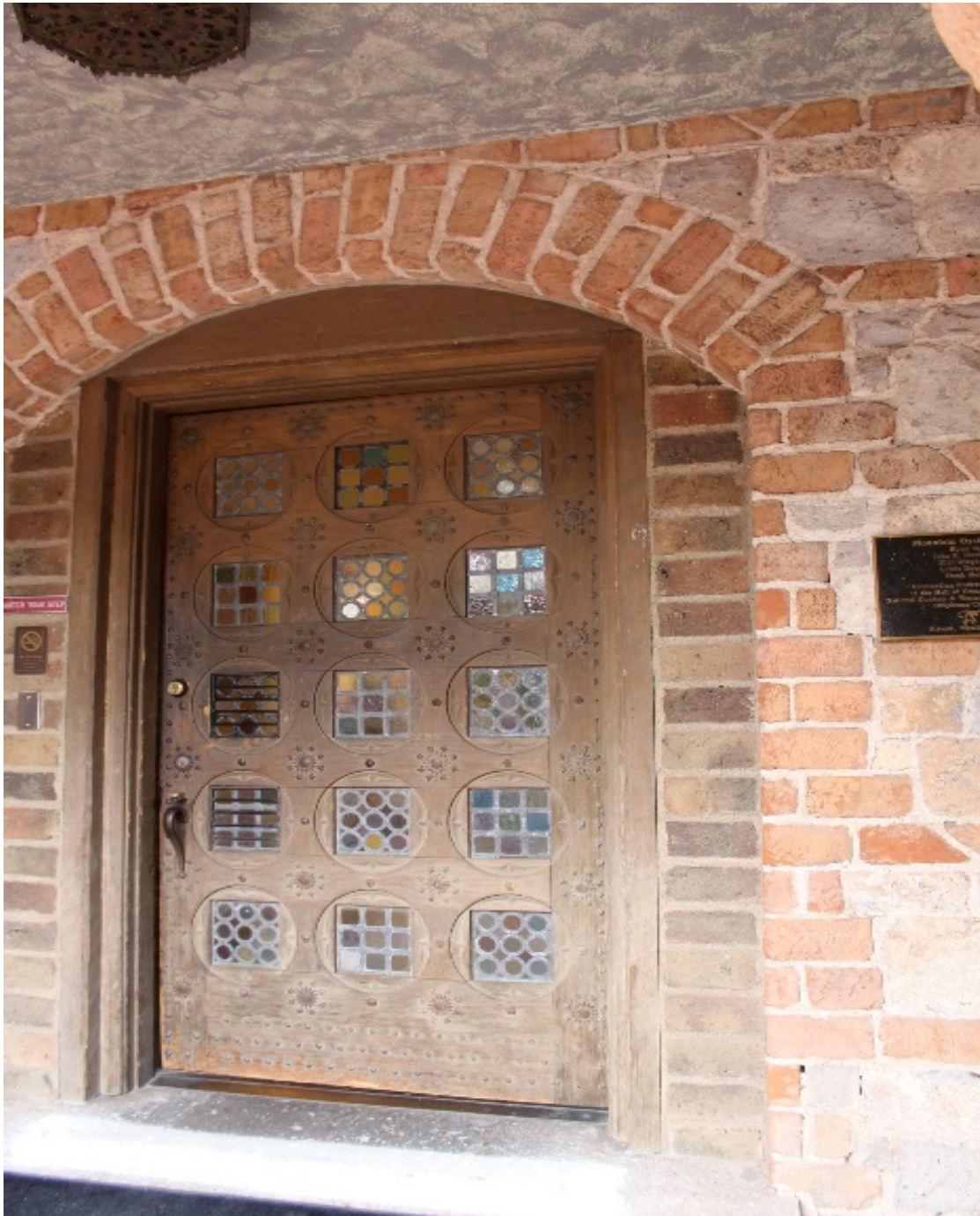
5 of 18. AZ_PimaCounty_ElDoradoLodge_0005 Hand-hewn Main Entry door of wood, iron and colored glass, Mountain Oyster Club. Facing East
