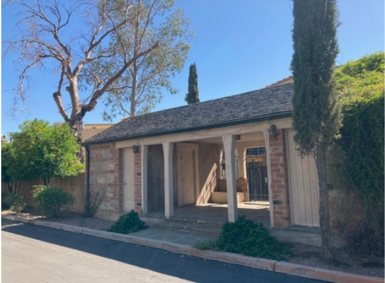
6 of 17 . AZ_PimaCounty_ElDoradoLodge_0006 Bathhouse on eastern perimeter of South Parking Lot, Mountain Oyster Club. Facing Southwest
