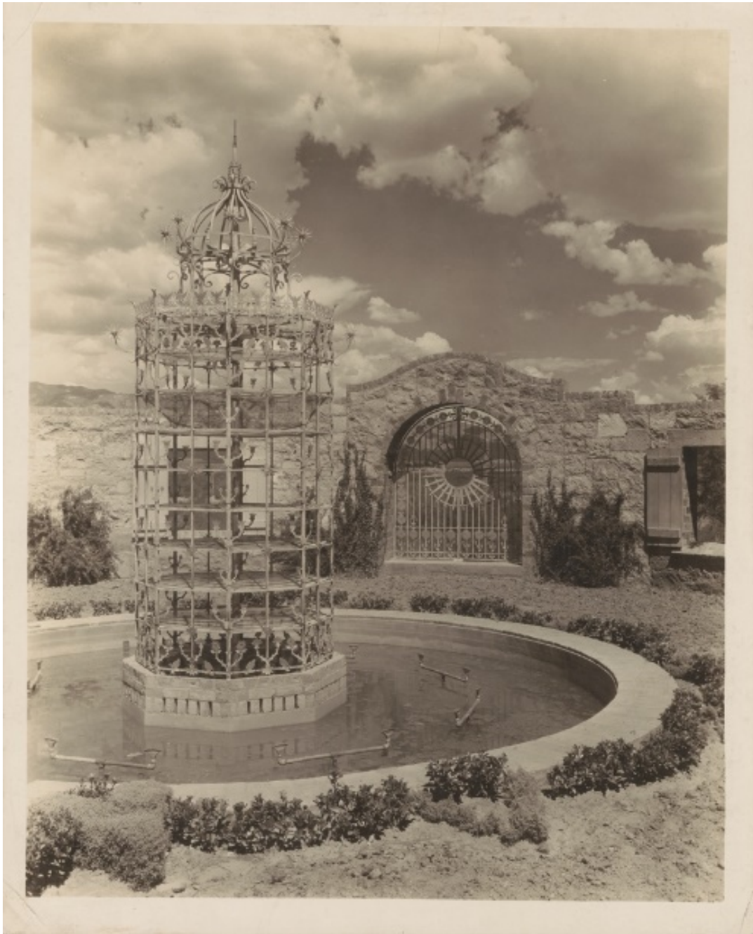
Figure 22. Original Wrought Iron Water-Cooling Tower, Circa 1946.
